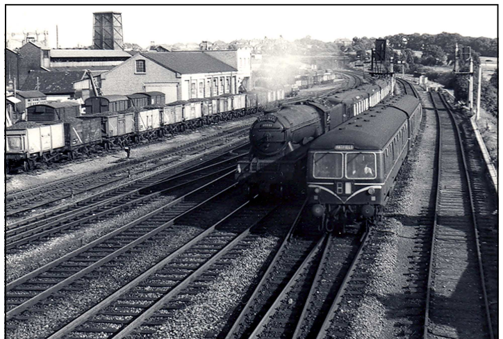
View southwards from footbridge at New Southgate Station
